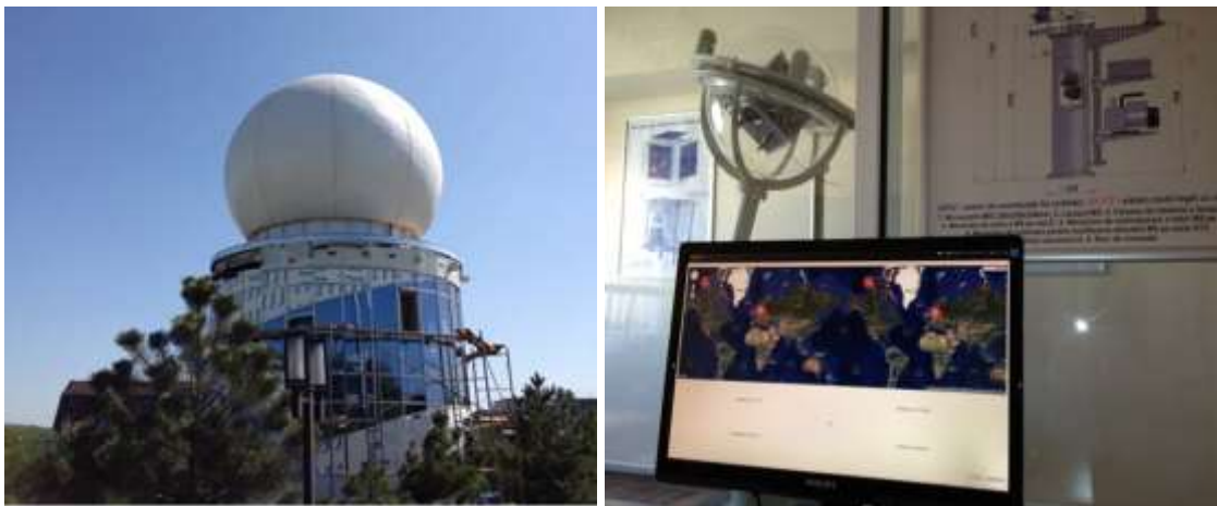
The ground station building and the software interface for satellites tracking.
